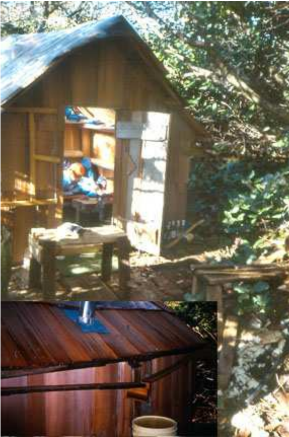
Deserters Cabin, showing the good effect of the plastic roof on interior light. Water catchment on rear roof at bottom
